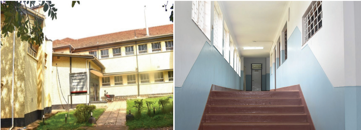
The renovated exterior and interior of the Department of Physics
