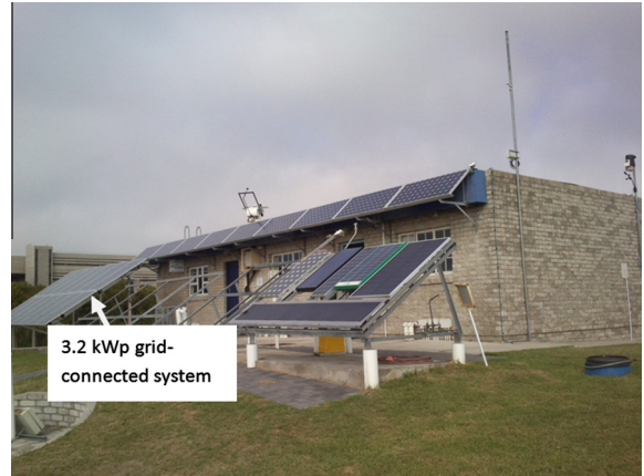
Fig. 1. View of the 3.2 kWp grid-connected PV system installed at the Outdoor Research Facility at NMMU.
